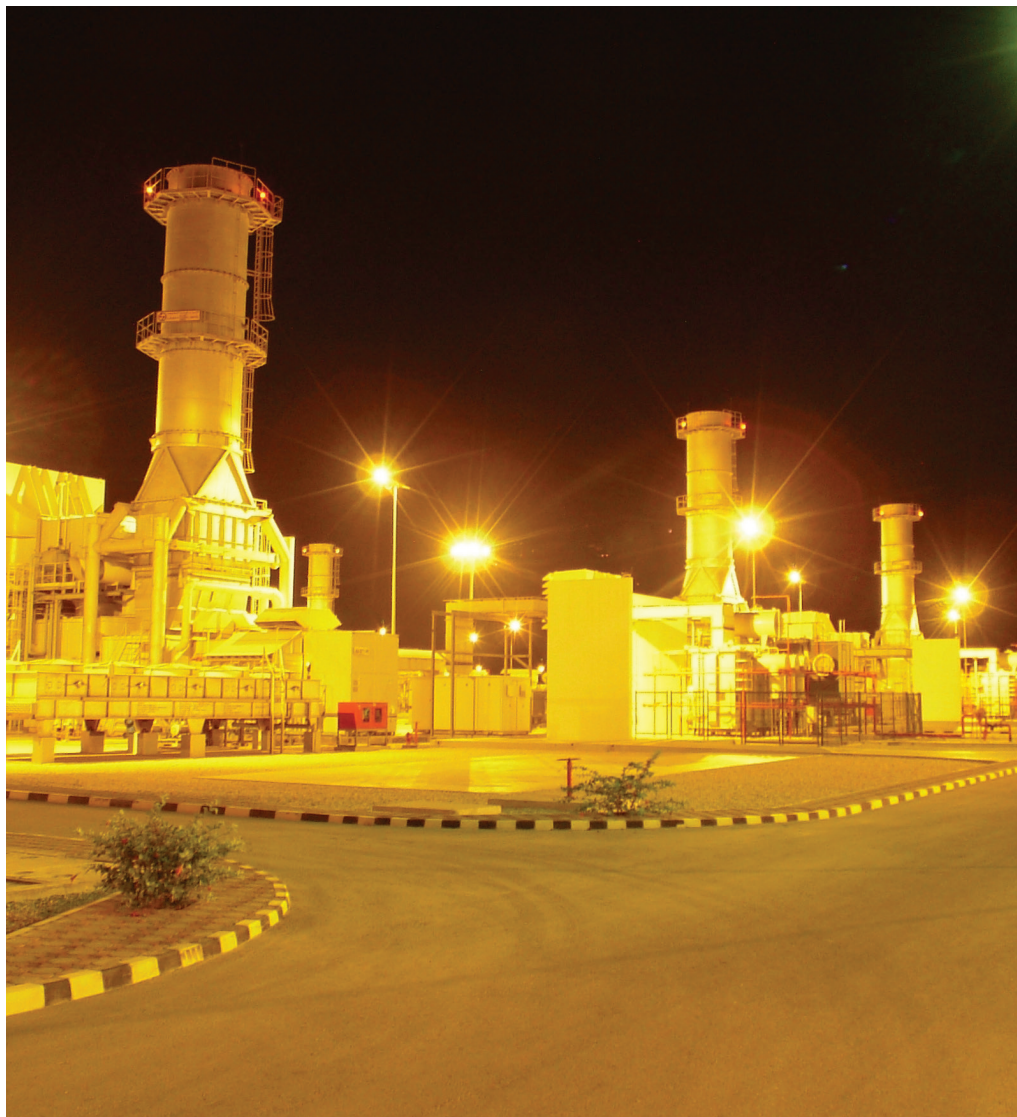
The existing plant
