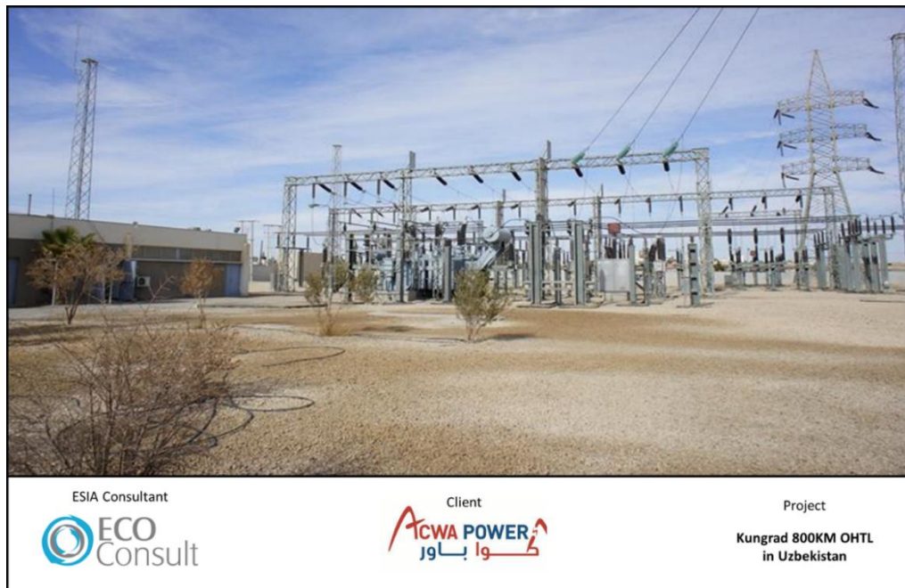
Figure 14: Typical Switching Station
