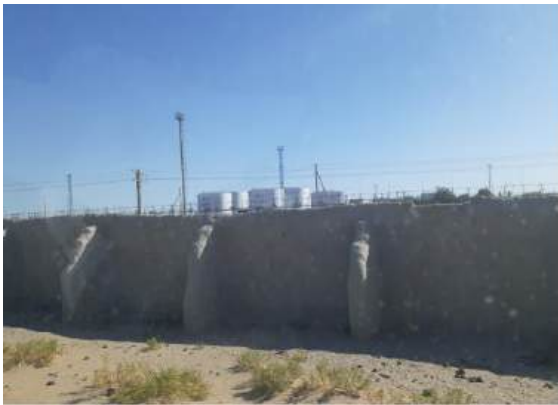
#R14– View of the Gas Storage Facilities from the Access Road
