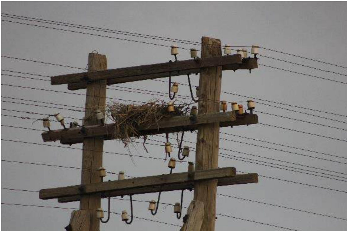
Plate 17-3 Common Buzzard's nest recorded on operating power line pole
