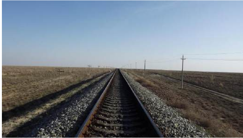
Plate 2-7 Railway Line crossing the Project site
