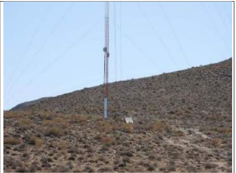
Figure 27 Cables holding the mast MM 6.
